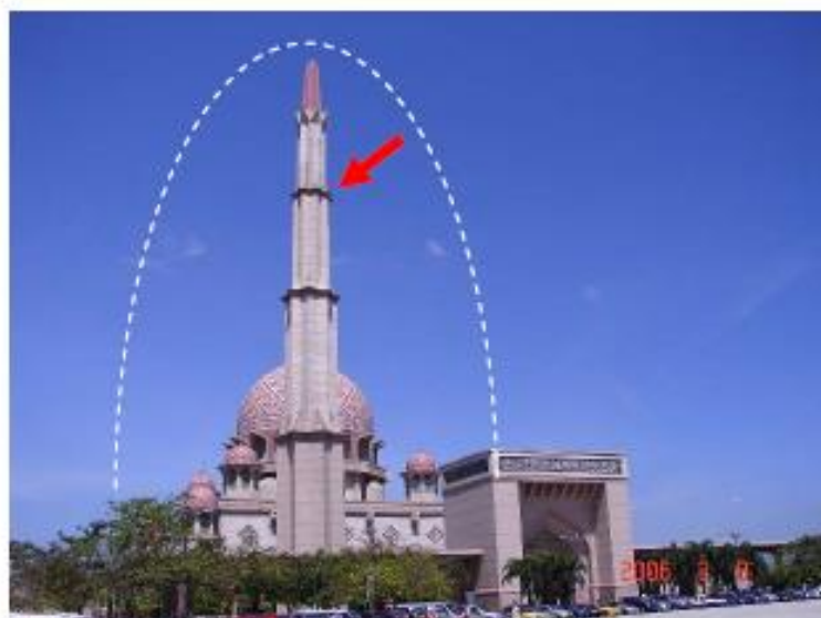
Fig. 5: Minaret of Putrajaya Mosque. The claimed protection zone is shown by the dotted line while the lightning strike location is shown by the arrow.
